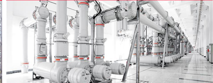
Gas-insulated substation
