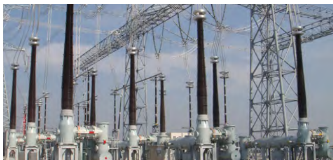
超々高電圧ガス絶縁開閉装置:UHV GIS (Ultra High Voltage Gas Insulated Switchgear)
